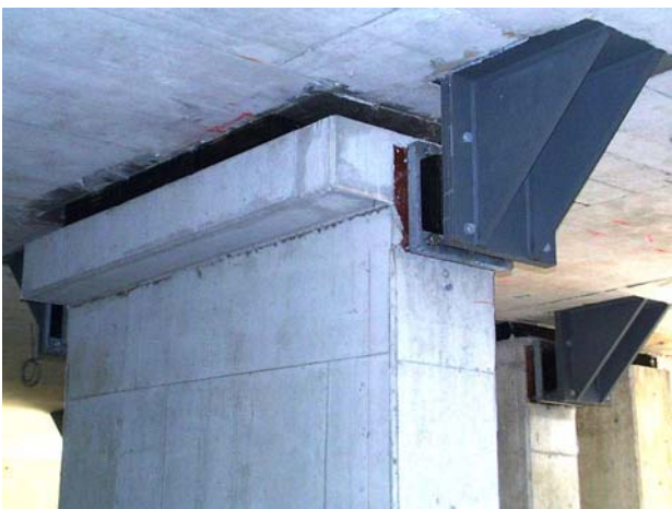
Figure 6 Town & Country condominium building isolation at top of garage level
