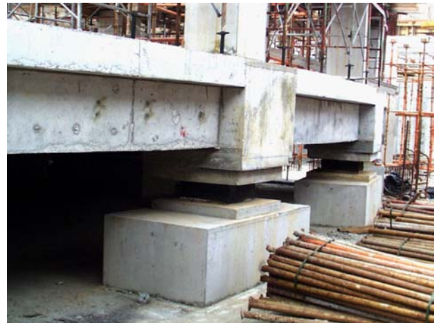
Figure 4 The Esplanade Concert Hall concrete structure at the isolation level
