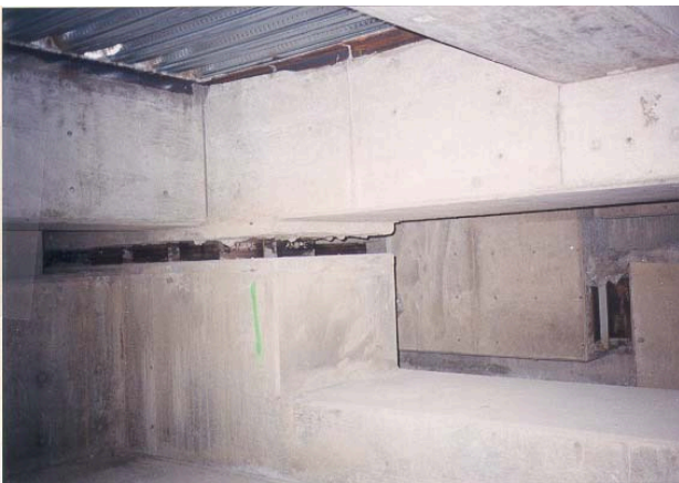
Figure 3 Benaroya Hall typical arrangement of concrete beams and bearing pads
