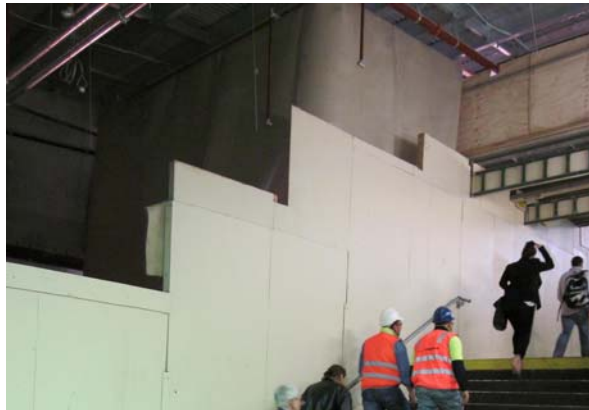
Figure 4. Temporary hoarding within underground station
