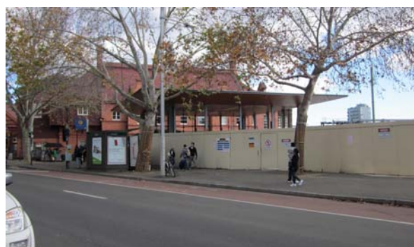
Figure 2. Temporary hoarding at station entrance
