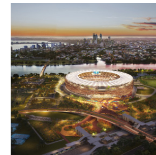
New Perth Stadium - WA
