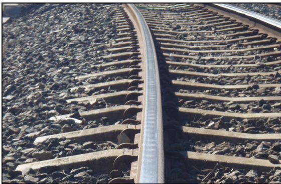
Figure 1. 9 month old corrugated rail profile
