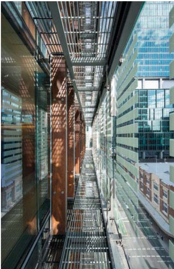
Figure 3 Vented or double skin facade
