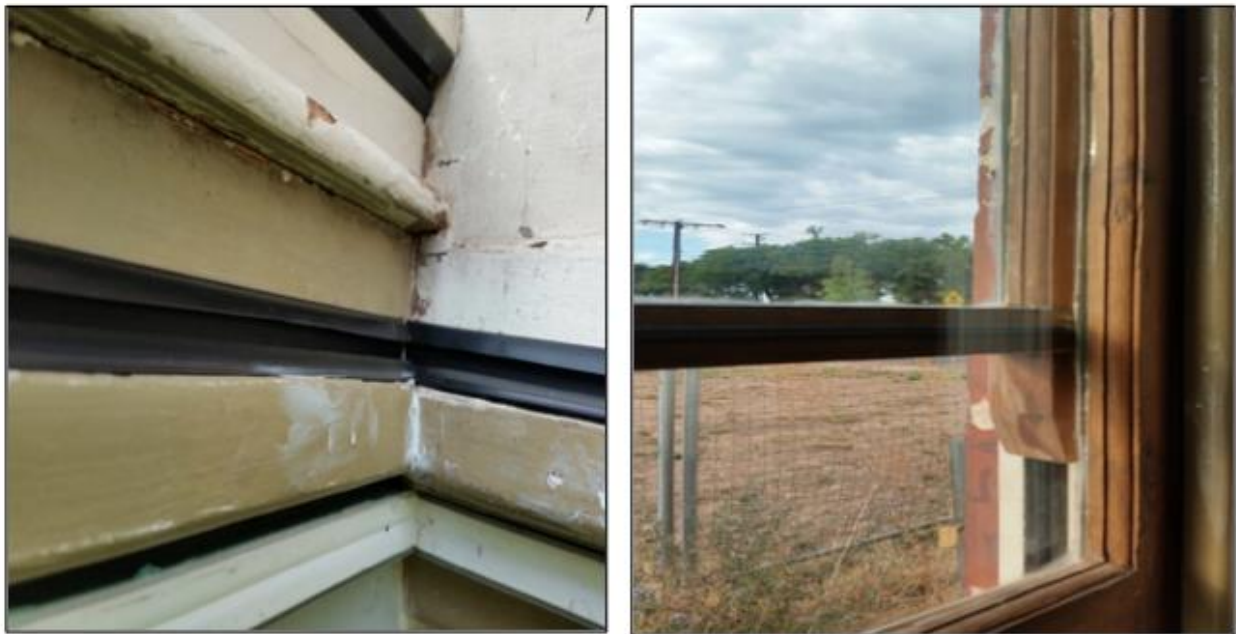
Figure 3. Raven RP 150 perimeter seals and laminated glazing
