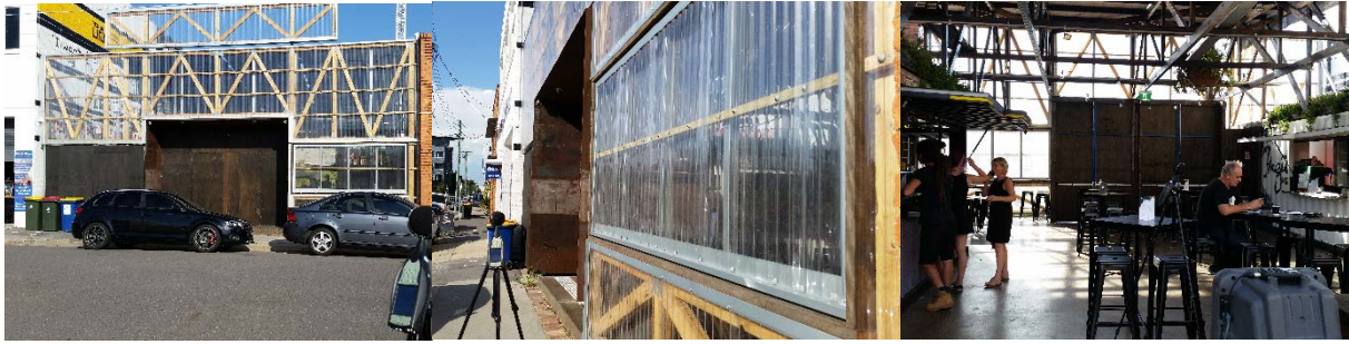
Figure 11. Lightweight polycarbonate noise barrier and roof system, beer garden
