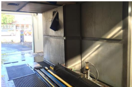
Figure 3: Car wash exit towards Camberwell Rd, with a residential house positioned opposite in the background
