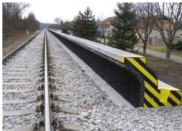
Figure 3 Low profile barriers sit on the ballast close to the track (from (Zvolenský, et al., 2017))
