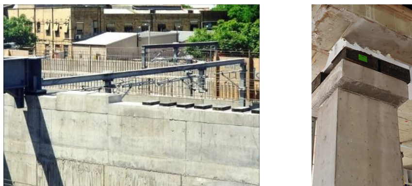
Figure 9: Natural rubber point bearings
