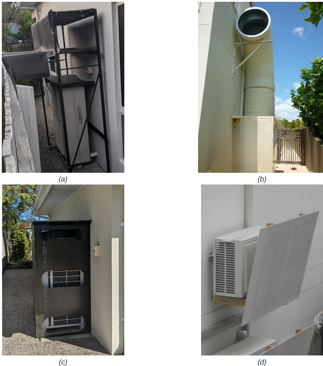
Figure 3 – Homeowner “solutions” to attenuate air-conditioner noise
