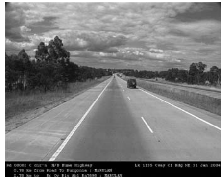
Photo 1. Section of highway (from Gipsicam)
