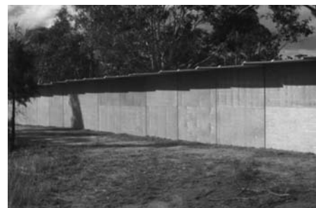
Photo 3. T-top barrier (2.4m)
